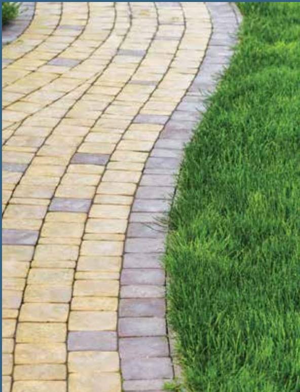
Correct Installation - Standard Edging
