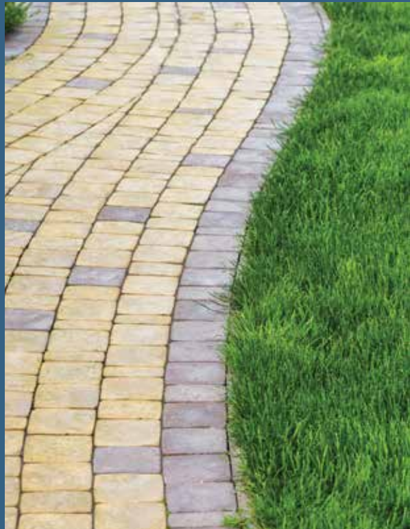
Correct Installation - Standard Edging
