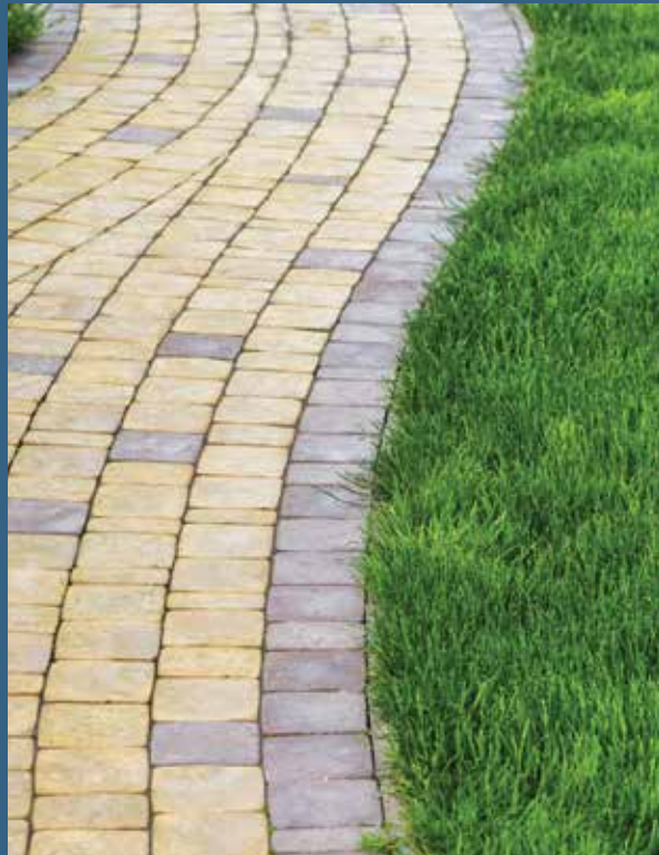
Correct Installation - Standard Edging
