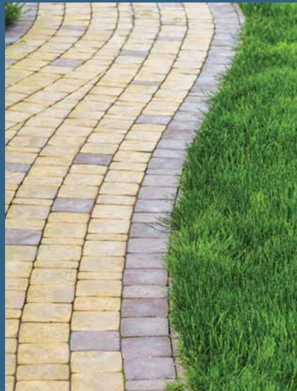
Correct Installation - Standard Edging
