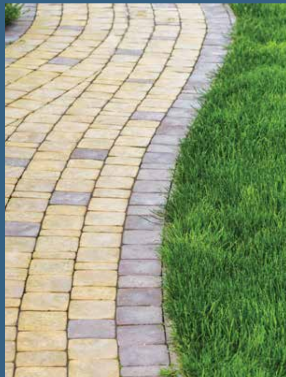
Correct Installation - Standard Edging
